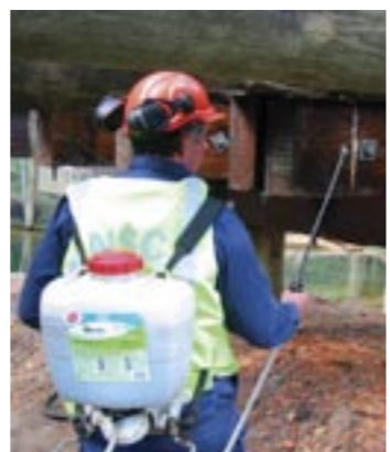
Spraying Lanolin Liquid on timber surface
