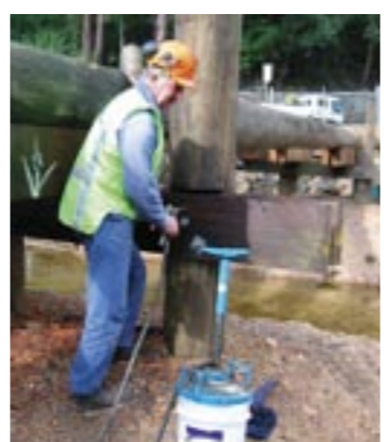
Pumping Lanolin Grease into timber joints
