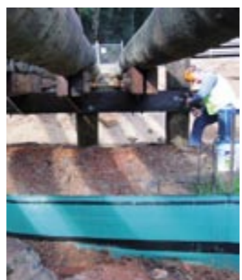
Pumping Lanolin Grease into timber joints
